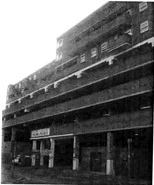
Bury Road Car Park
